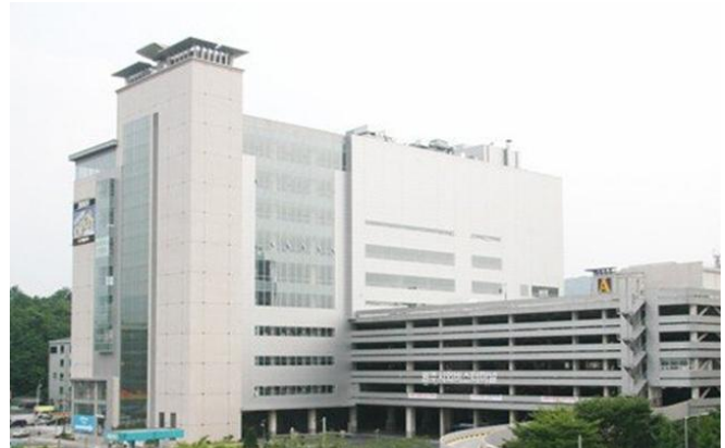
● Wonju Cross-country Bus Terminal Building
